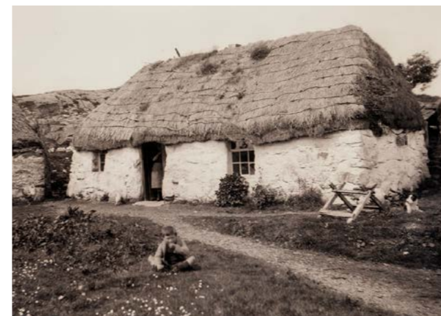
Thatched cottage. Duncan MacPherson Collection. © Highland Archive Centre
